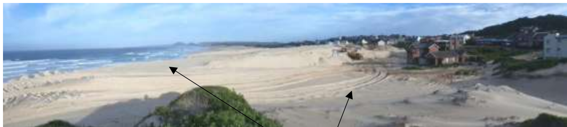
Foreground pushed already. Background and to the right still to be pushed back.
